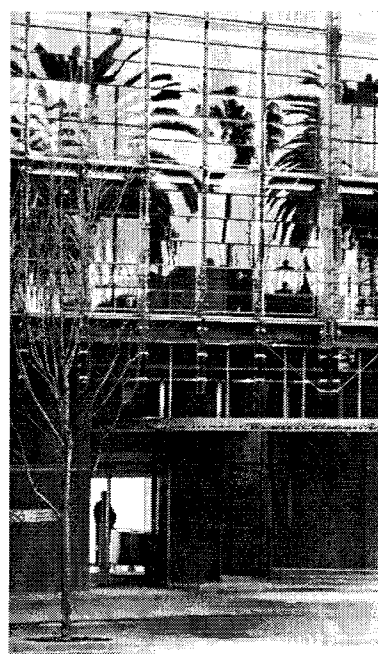
Fig. 13. Main facade detail. Residential block.
